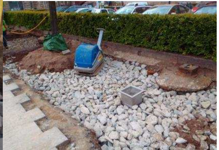
Recycled concrete used as a part of the structural soil instead of granite
