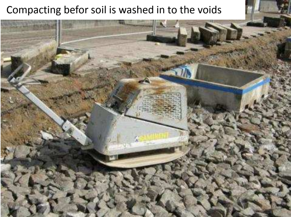
The stone shall fall into the box to get a stabel construction
